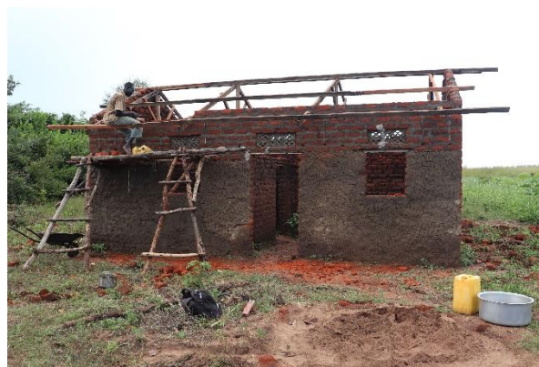
Mr. Aluma's 6 Meter by 4 Meters permanent house under construction
